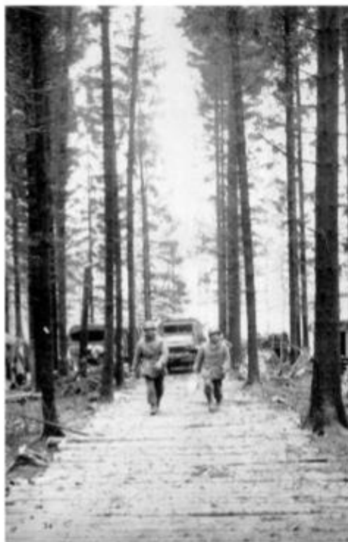
New roads had to be cut through the trees and paved with logs so trucks could move up
